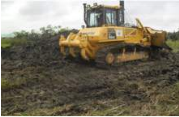
Excavator at work and consultant inspecting the work of the excavator
