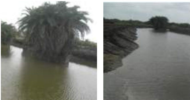
Plate 5: Dredged Ntakofam River at completion
